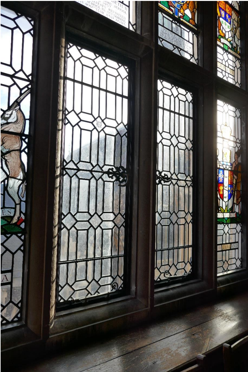
Close up of part of window concerned.
